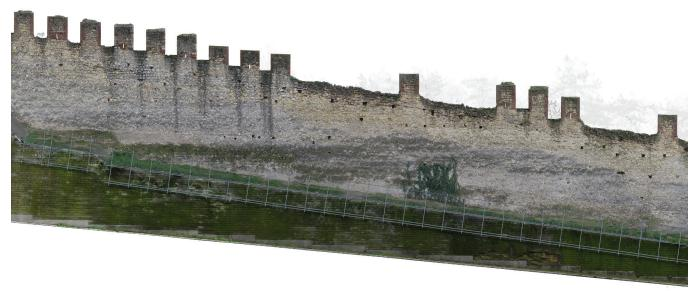
Fig. 7 – Example of high-reliability close-range and ground-based photogrammetric techniques. This type of processing was carried out for the entire length of the wall section (600m).
