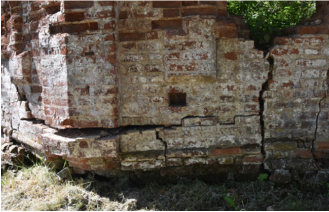
Fig. 1 The shape derived from structural damage to Built Heritage is recognisable, and defines a distinct morphometric character both as a crack and as a continuous deformation. For a reliable digital form to perform structural simulations, the detail of 3D acquisition and representation becomes central. Above, local crack conditions in a historic masonry structure; right, 3D polygonal mesh digital surface of a crack with detachment on a structural surface.
