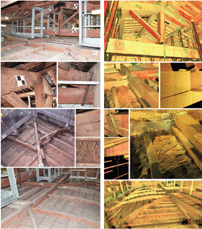
Fig. 1 Digital survey of a 'canniccio' vault and its wooden structure in the Uffizi museum complex. Photographic survey (left) and 3D point cloud views (right).
