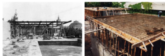
A concrete slab was chosen instead of a metal profile structure. The bituminous fabrics were replaced by waterproofing grey polyester. The overall layout of the slopes was modified. Six drains were added, non-existent in 1929
