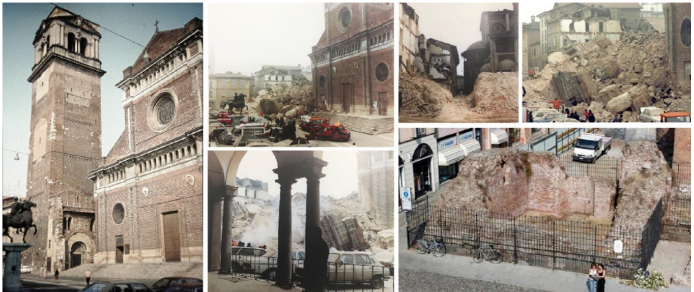
Fig. 5 Collapse of the Civic Tower of Pavia in 1989. The absence of monitoring activities on the historical structure did not evidenced the crack conditions and damages.
