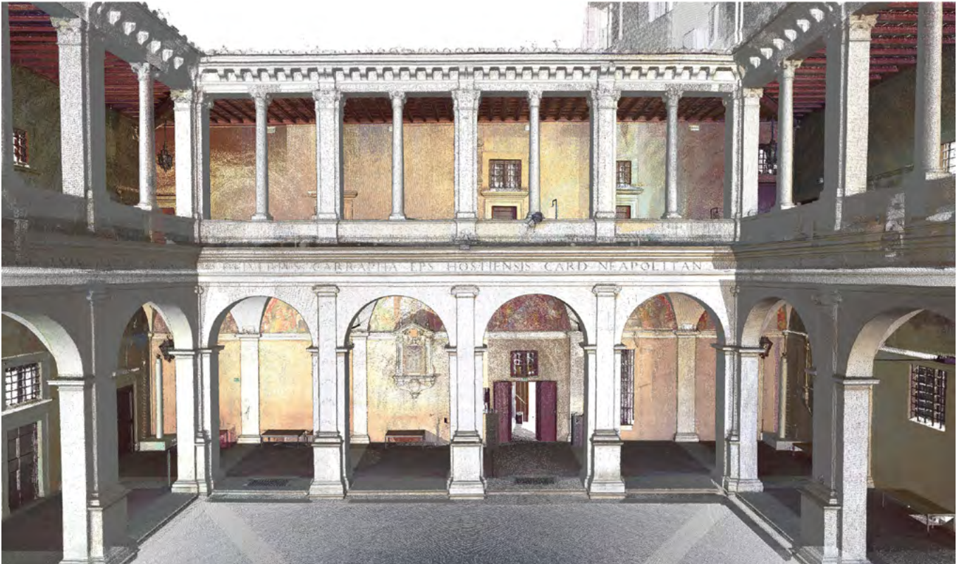
Fig. 1 - The cloister of Santa Maria della Pace. Laser scanner point cloud visualization.
